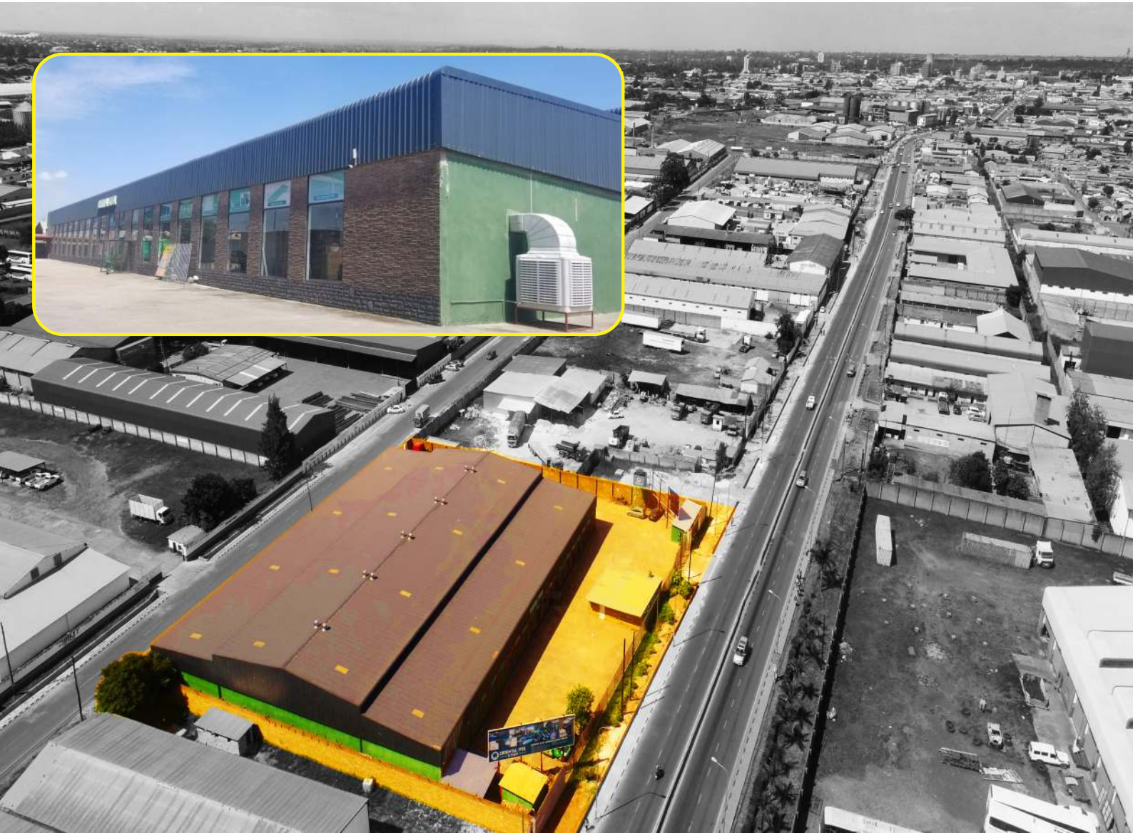
Sales Outlet and WareHouse
